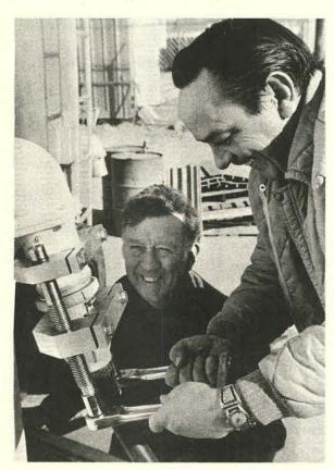
NEW TOOL — Leo Dunn (1914) and Gerry Hastings (9655) demonstrate how their device disconnects mated cable connectors on an instrumentation van. Clamps, threaded shafts and two ratchet wrenches linked at the handle make it possible to apply straight line force of several hundred pounds on the two parts of the connector.
